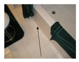
It is recommended to caulk the gaps between the tile floor and tub in the upstairs hallway bathroom to avoid moisture intrusion into the flooring.
