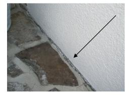
Moisture intrusion was noted around the outside band in the crawlspace behind the front porch. It is recommended to seal the gaps between the stone and front wall to avoid further moisture intrusion. Repairs were noted in the outside band behind the front porch.
