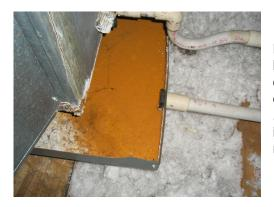
Rust stains were noted in the drain pan below the upstairs air handler. This is often an indication of problems with the cooling unit. The outside temperature was too low to run the cooling cycle at the time of inspection. This unit appears to be 17 years old. It is recommended to have the upstairs HVAC unit inspected by a qualified HVAC technician with repairs/replacement made as needed.
