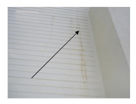
Stains were noted on the left wall behind the chimney. No moisture was noted in the stained areas on the lower section of the wall. This area should be closely monitored with repairs made as needed. (This is on the outside wall behind the master bathroom sink. The plumbing supply and drain lines terminate through the exterior wall.)
