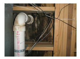
Moisture stains with soft wood was noted in the sub-flooring below the downstairs bathroom toilet. Further investigation is recommended by a qualified plumber with repairs made as needed.
